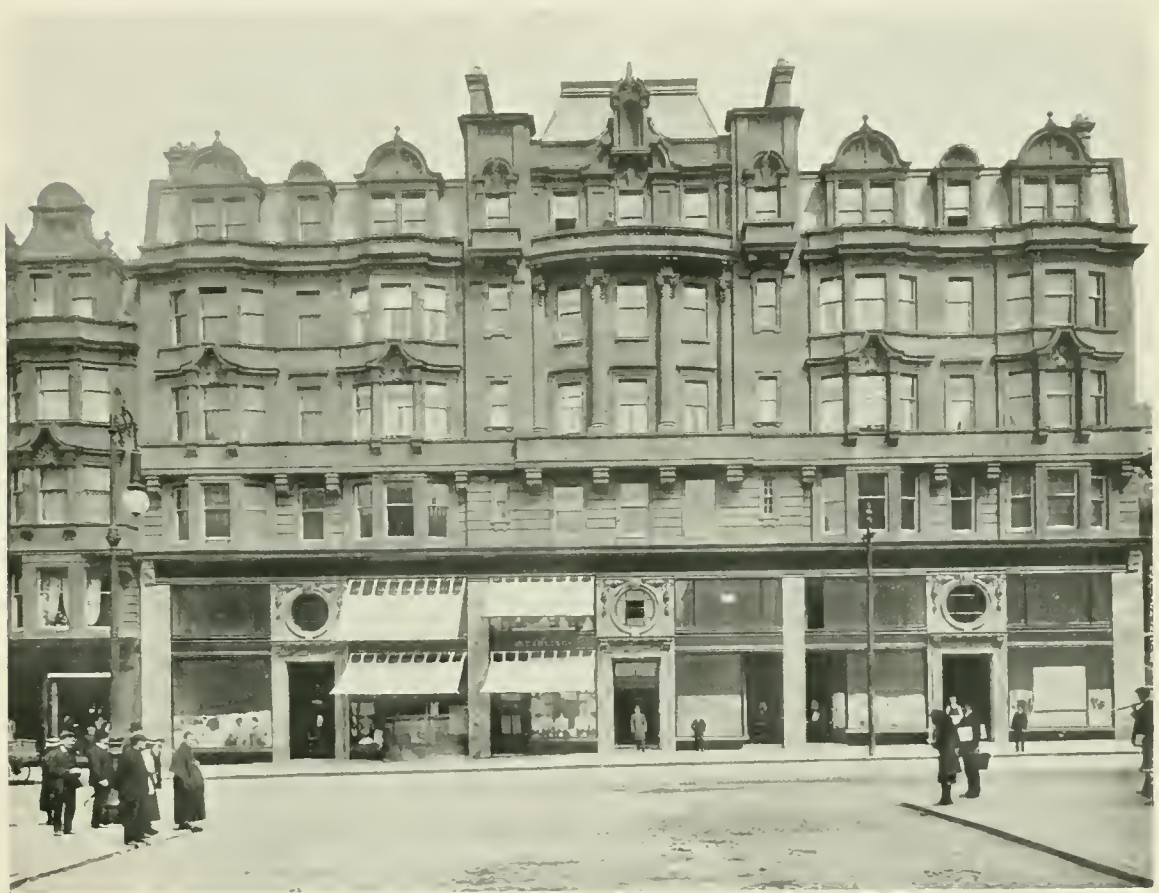
SHOPS AND RESIDENTIAL FLATS IN SAUCHIEHALL STREET, GLASGOW. THE FRONTAGE IS 330 FEET. SEE THE PLAN ON THIS PAGE. THE FLATS ARE LET AT £70 A YEAR, AND THE SHOPS AT RENTS VARYING FROM £150 TO £300
